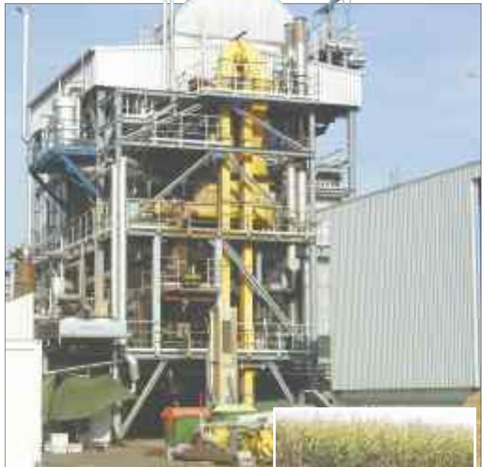
ENERGY ECONOMICS (above): Gussing biomass plant which produces 2000kWh of electric power, plus 4500kWh for district heating.
